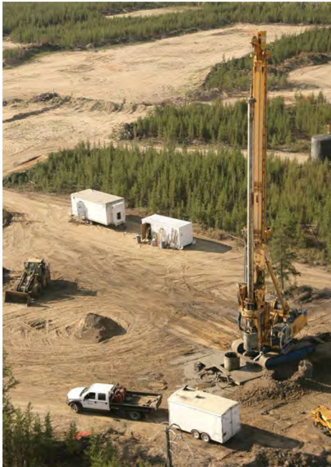
FIGURE 5. LDD rig in Kelly drill mode (note casing and support equipment)
