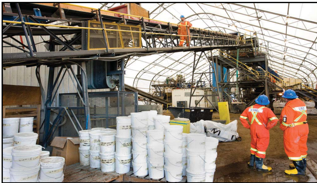
Onsite Processing Plant interior
