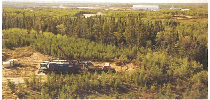
Angled core drilling for the protection of ravine environment
