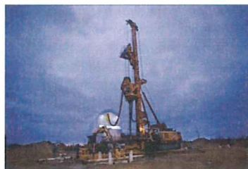
Bauer 1.2 metre large diameter drill
